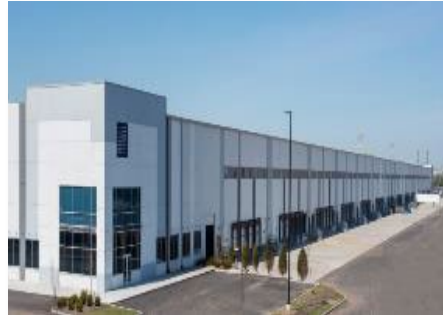
586 Gulf Avenue, Staten Island, NY
